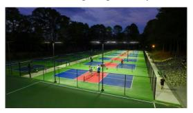
Lighting. Designed specifically for the court, Baseline uses a Type IV CL precision optic designed especially to meet IESNA / USA Pickleball / USTA Standard Performance Criteria for court photometrics. The luminaires distribute uniform light across the court surface without creating hot spots. To minimize glare, the light is directed at a low angle onto the court surface avoiding direct glare into the eyes
